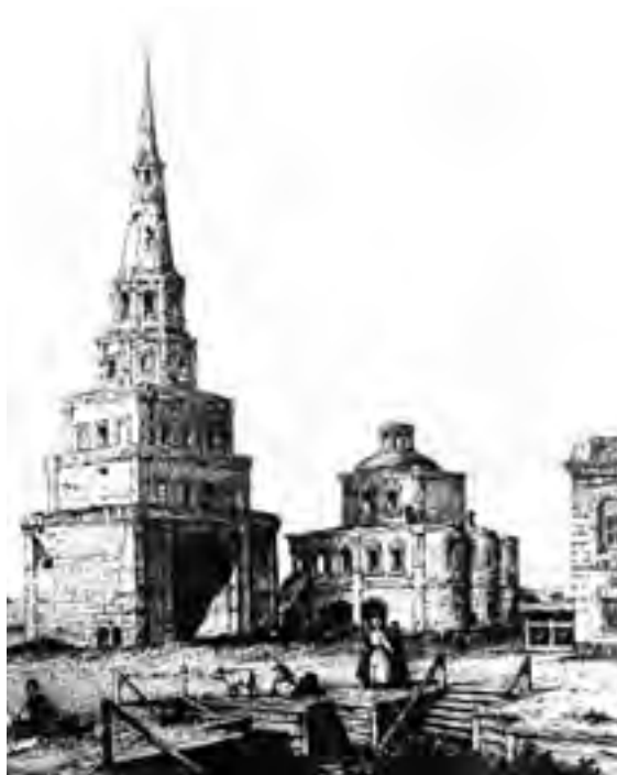
Fig. 10.62. The Sumbeki (Syuyumbeki) Tower in the Kazan Kremlin. From the drawing by Edward Turnerelli. First half of the XIX century. Taken from [944], p. 731.
