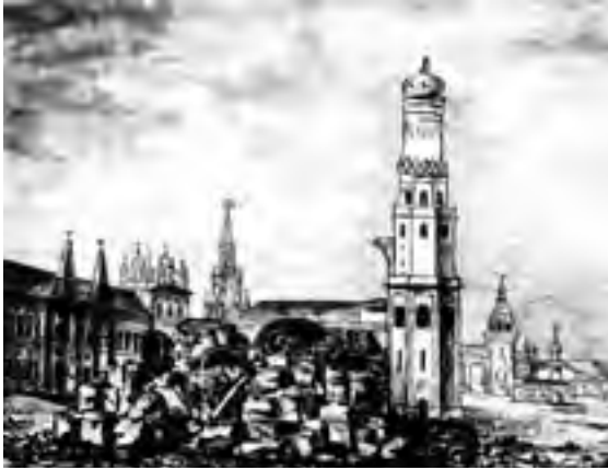
Fig. 10.58. View of the Ivan the Great Bell Tower and the annexe to it destroyed by the French in 1812. “Ivan the Great’s bell tower remained unharmed (it only cracked). The Petrok Maly Belfry and the Filaret’s Annexe turned into ruins” ([96], ill. 89). Drawing by architect A. Bakarev. Taken from [96], ill. 89. See also [283].
