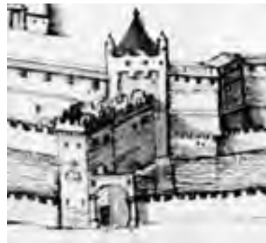
Fig. 10.15. The Kremlin’s imposing Timofeyevskaya gate tower. Image from the early XVII century plan. Note the triple walls surrounding the Moscow Kremlin. Taken from [773], p. 23.
