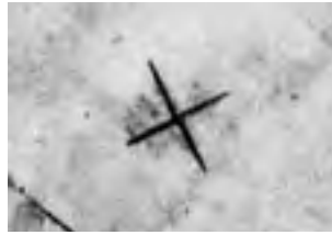
Fig. 12.29. A small cross on the stone floor of the Great Sofia. These crosses mark the projection of the dome’s circumference. They were made during the construction of the dome. Taken from [1123], p. 14.
